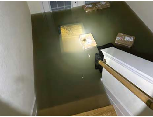
Water rises in a home on the barrier islands.
