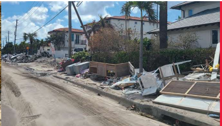
Debris lines both sides of Gulf Boulevard following Hurricane Helene.
